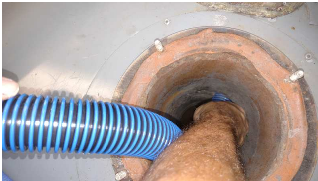
Hose Inserted into Swirl Tube Heat Exchanger
