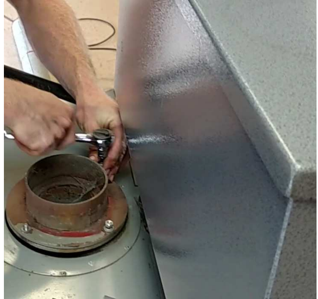
Flue Tube Assembly Bolted Flange
