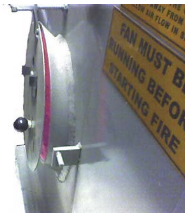
Sight Tube Cover in Open Position
