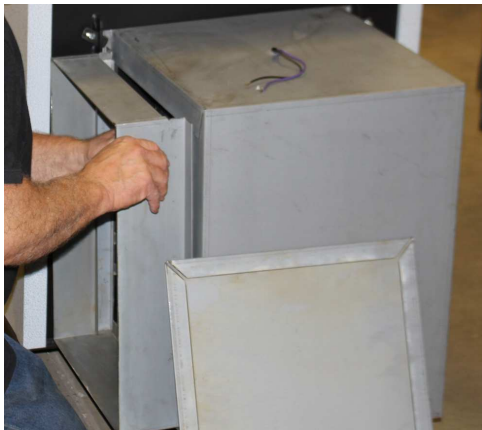
Installing Filter Rail
