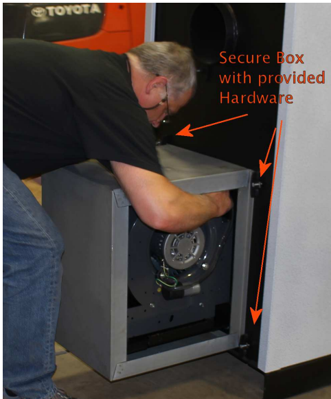
Securing Filter Box
