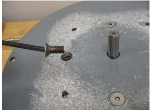
Closeup of Motor Mounting Bolts
