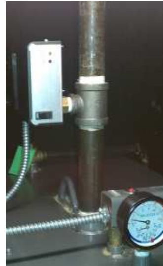
Photo: Low Water Cutoff Installation
