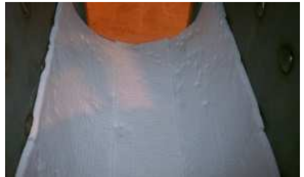
New Ceramic Blanket in Place
