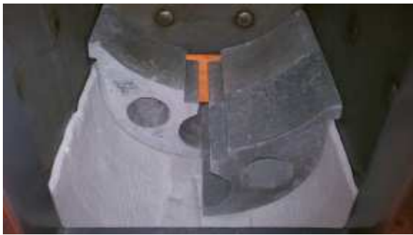
Positioning New Side Brick
