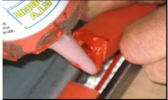
Adding High Temperature Silicone to Butt Joint of Trimmed Bead
