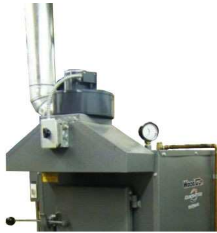
Smoke Hood Installed
