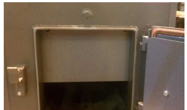
Photo: (Smoke flap installed)
